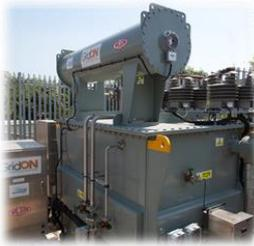
GridON's breakthrough fault current limiter (FCL), which suppresses the damaging currents resulting from electricity network faults, has successfully completed its first year of operational service on UK Power Networks' primary substation at Newhaven, East Sussex, proving both reliable operation and extremely effective performance in limiting several network fault events.
